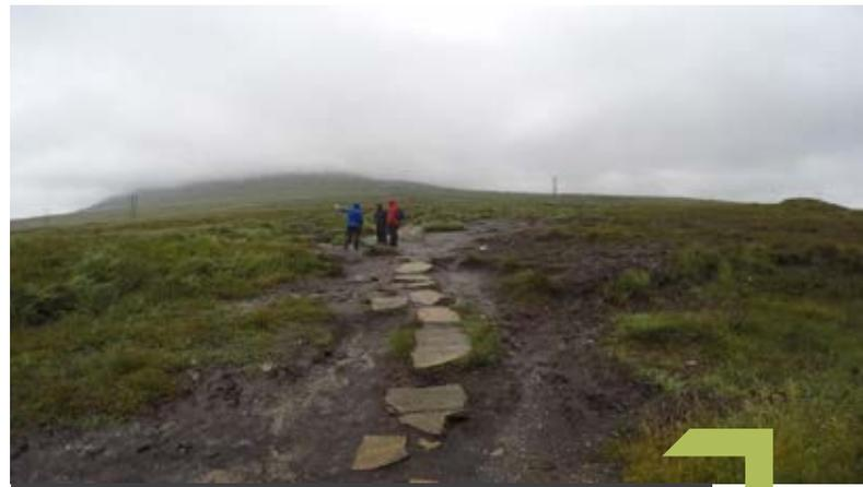
Figure 2: Trail Access from car park to Direct Ascent Route displaying attempts to pave path and erosion damage.
